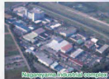
Nagareyama industrial complex
